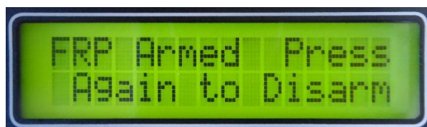
Figure 5 - Message indicating that Factory Reset is armed
